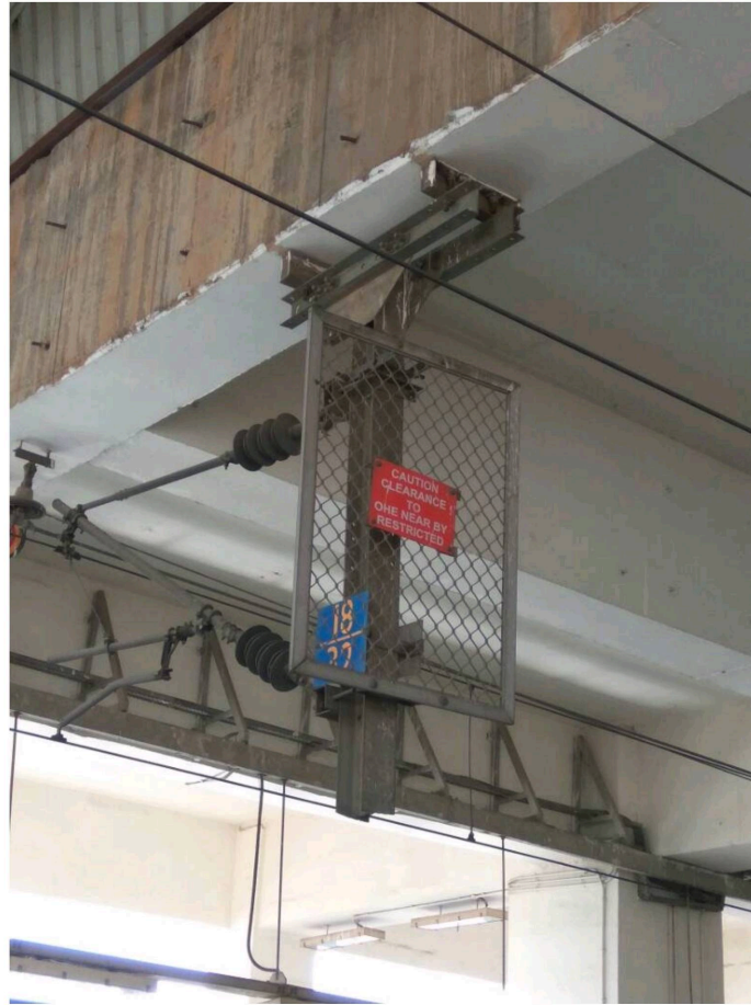
Figure 11: OHE suspension arrangement at DMRC's Tuglakabad station (1)
