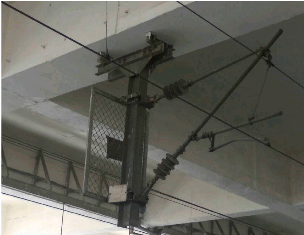
Figure 13: OHE suspension arrangement at DMRC's Tuglakabad station (3)
