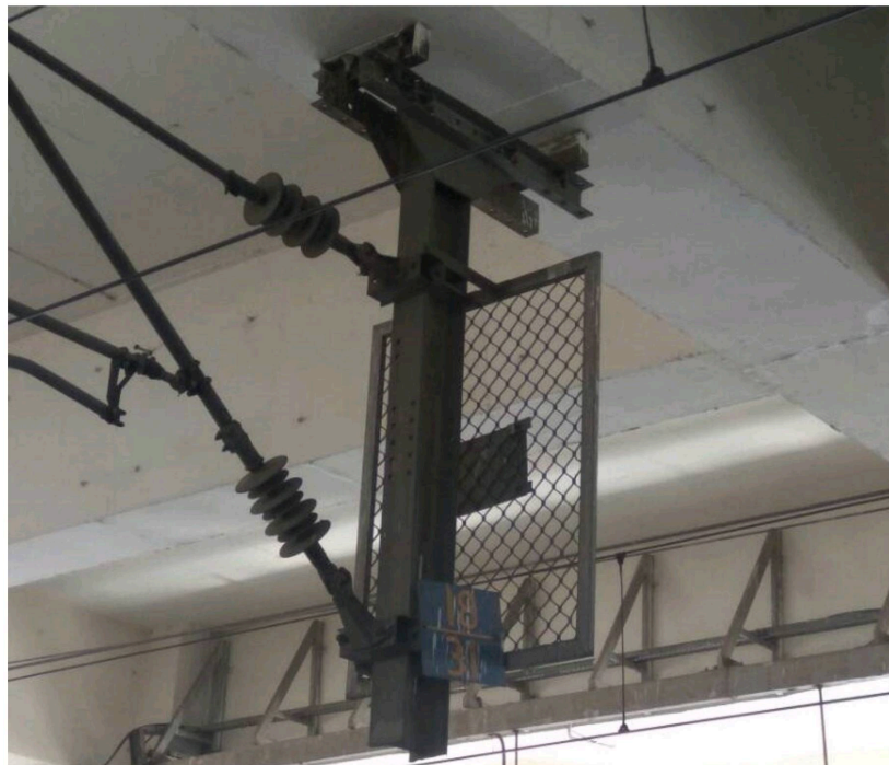
Figure 12: OHE suspension arrangement at DMRC's Tuglakabad station (2)
